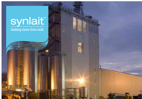
Dunsandel, Canterbury Upgrades $204m + $125m
